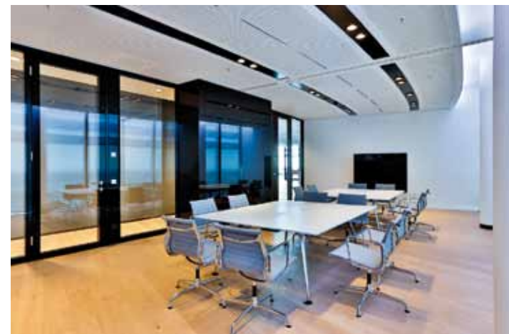
On the 18th floor, structural glazing walls fitted with black bonding and with surface-flush 100 mm doors create a design highlight.
