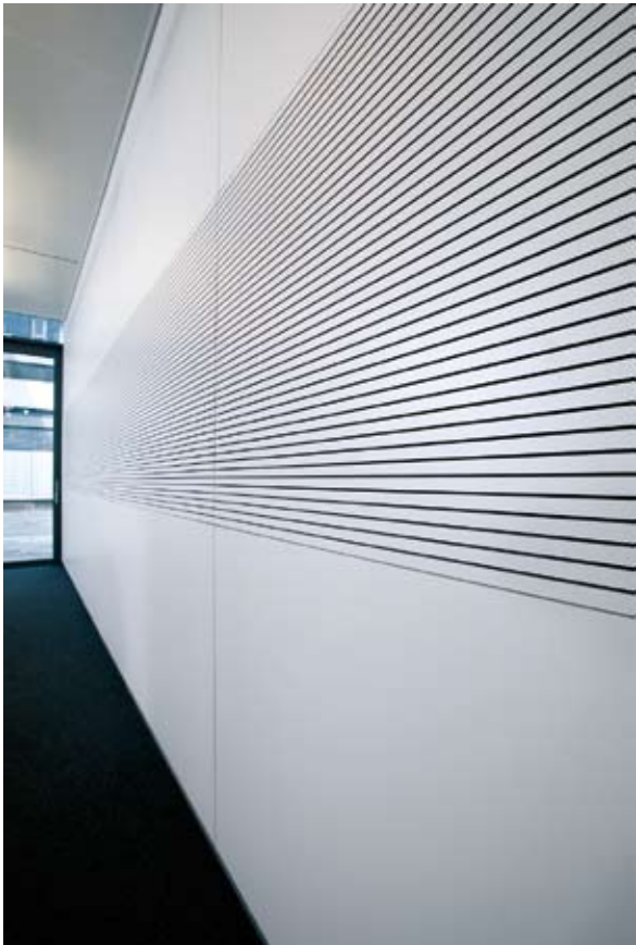
Flush-integrated partition wall absorbers, together with absorbers on the ceilings and on the exposed concrete walls, as well as freestanding absorbers in the open-plan offices are all from the 7000 system and provide the quiet needed for concentrated working.
