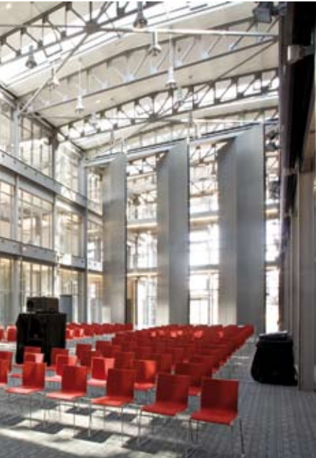
The atrium in the conference centre extends over three storeys. Glass partitions, 125 mm thick, fulfil the static requirements. The large element dimensions demanded an individual fire safety testing for this project which the system 2300 passed successfully in accordance with the Swiss fire rating standard R30 (equivalent to the E30 standard).
